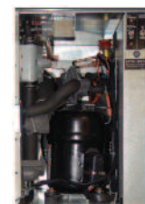
Dry Electrical and Compressor Compartment
